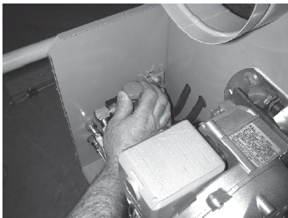
Close the fuel line shut-off valve
