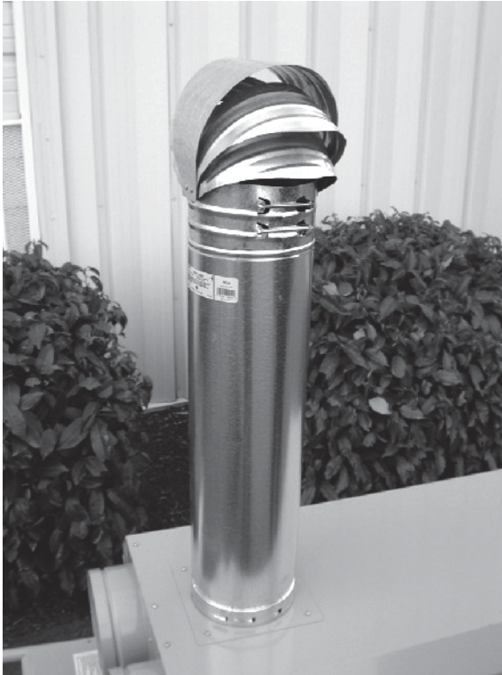
Attach the flue to the Dragon
